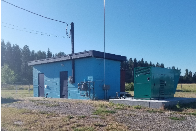
Lodge Road Pump House
